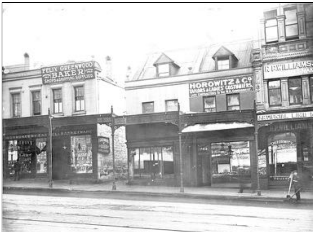
Figure 12: South-east facing view of 751 to 759 George Street in 1910 (NSCA CRS 51/302).
