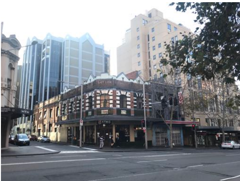
Figure 29: The Site. Nos 761-763 and 757-759 George Street.
