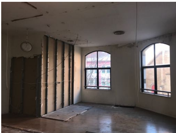
Figure 45: Nos. 761-763 George St First Floor interior.
