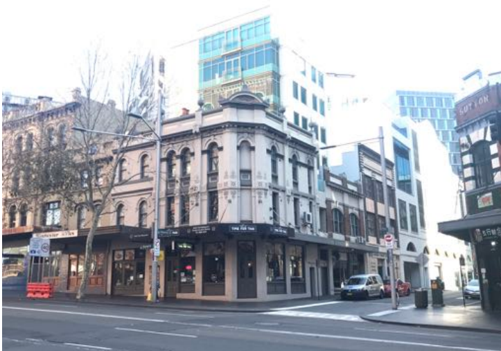
Figure 52: Commercial Building group including interiors. Nos. 767-791 George Street, Haymarket, Sydney. (1844).
