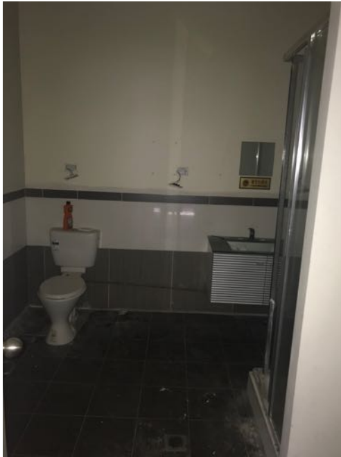
Figure 46: Nos. 761-763 George St First Floor interior.
