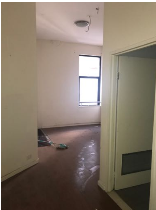
Figure 47: Nos. 761-763 George St First Floor interior.
