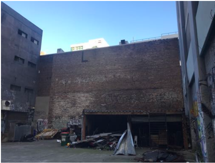
Figure 38: The Site, parking lot.
