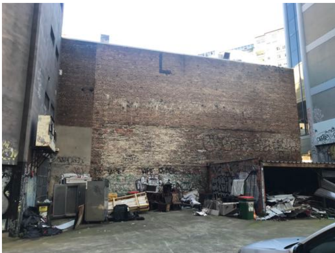
Figure 39: The Site, parking lot.
