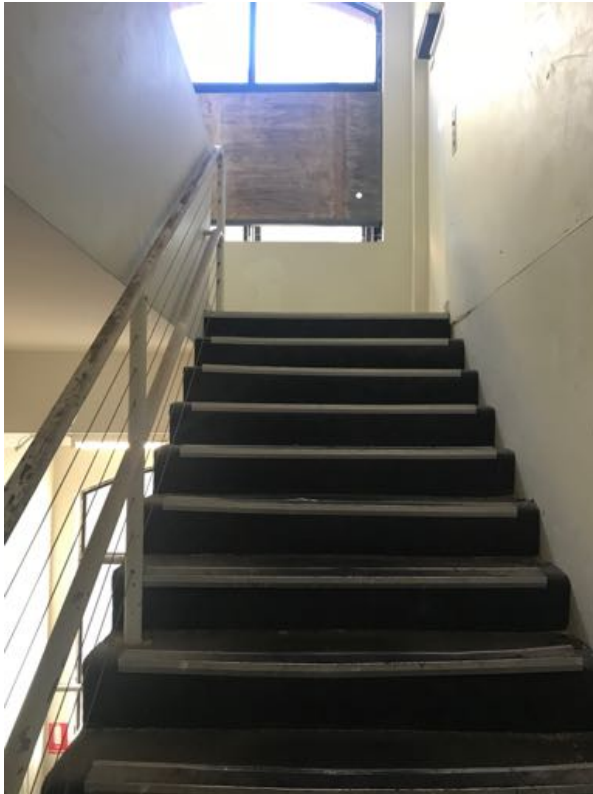
Figure 43: Nos. 761-763 George St stair up to first floor.
