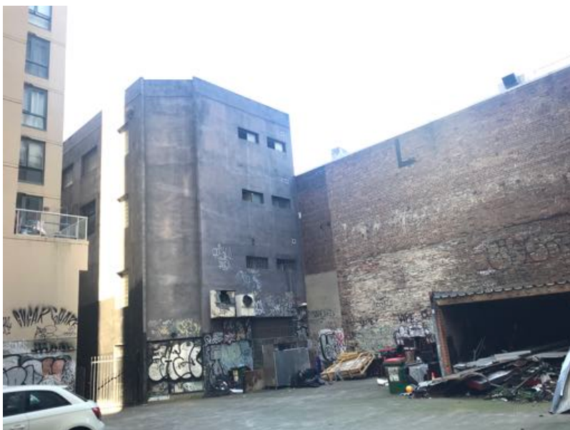
Figure 49: Nos. 757-759 George Street. From the rear parking lot.
