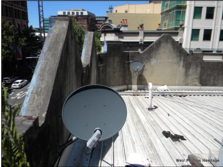
Figure 40: Nos. 761-763 George St - roof.
